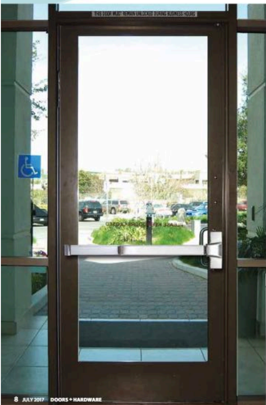
Single-door electric push bar and ADA bollard
