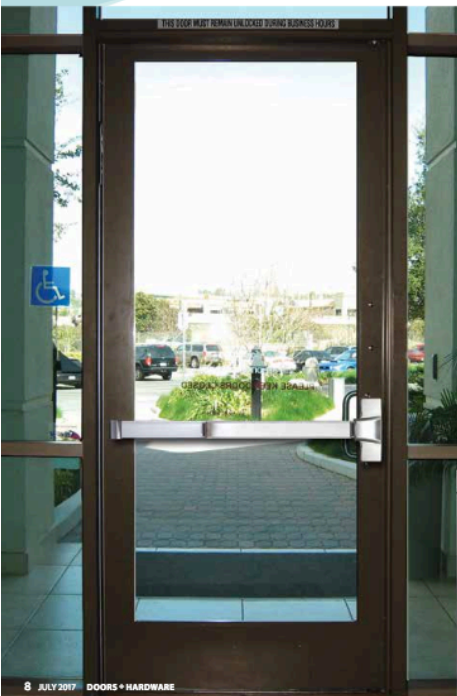
Single-door electric push bar and ADA bollard
